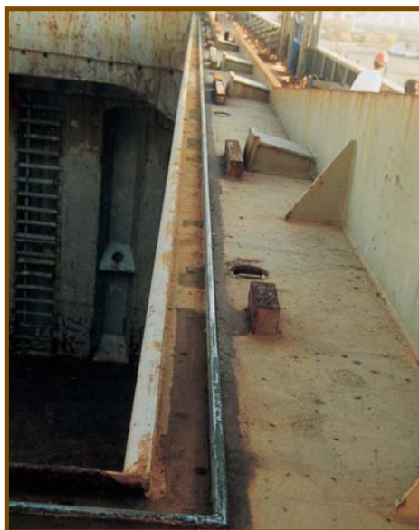
The double drainage system.
